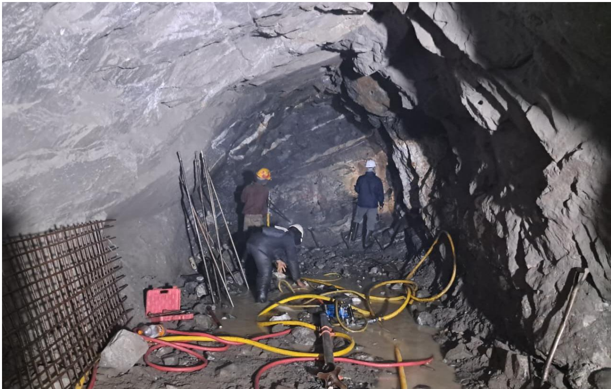
Figure 6: Drilling work in Inlet tunnel at ch 0+090.65m
