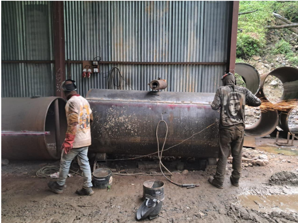
Figure 17: Grinding for welding in straight pipe in HM workshop
