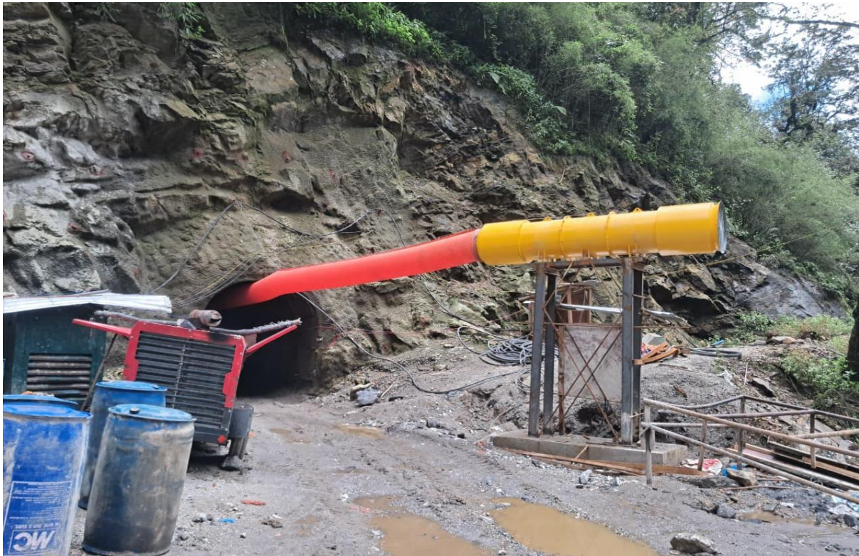
Figure 7: Ventilation installation in Inlet tunnel
