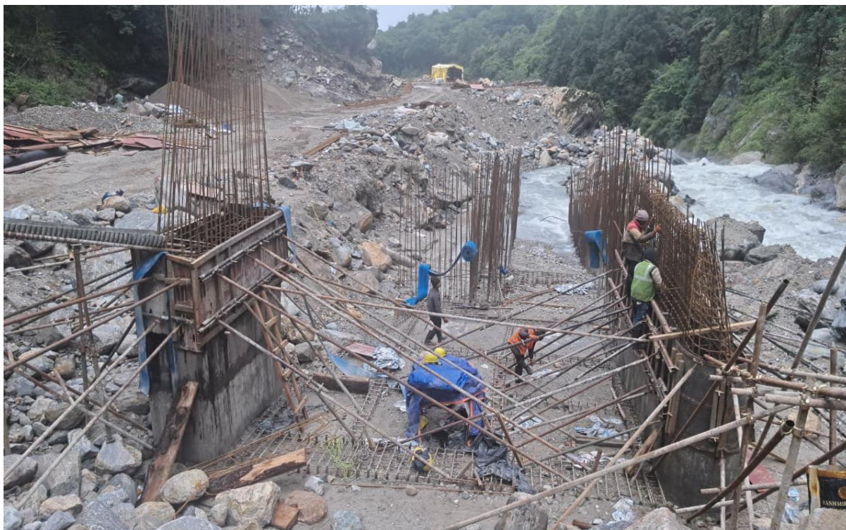
Figure 1: Preparation for concreting in wall of Undersluice u/s panel
