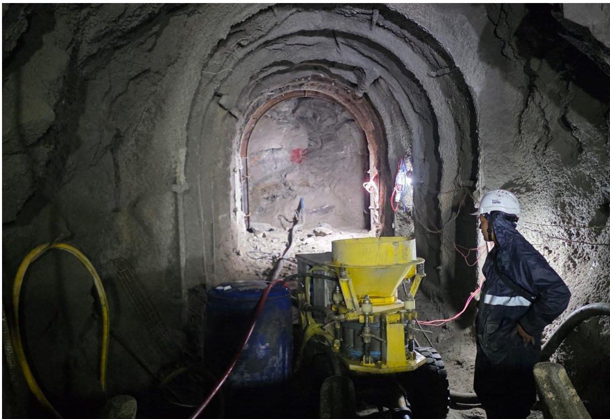
Figure 4: Preparation of shotcreting in Inlet tunnel
