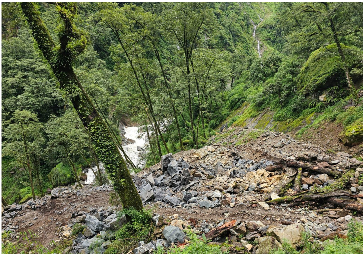
Figure 13: Drilling blasting in boulders in penstock alignment for road alignment near switchyard
