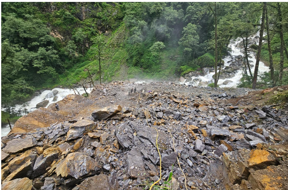
Figure 14: Powerhouse area after blasting
