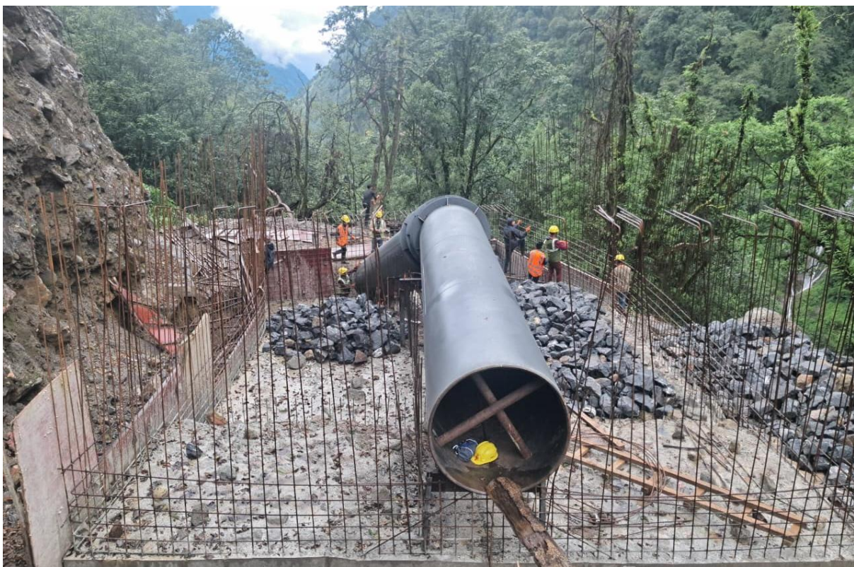
Figure 8: Rebar work in AB 12
