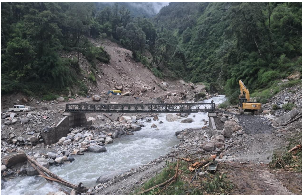
Figure 10: Bailey bridge installation in Nyadi river towards Powerhouse Road
