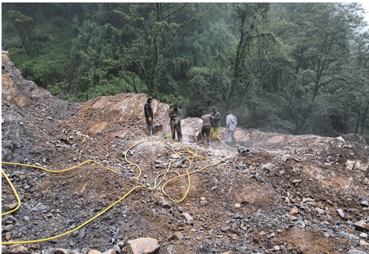
Figure 12: Drilling in powerhouse area
