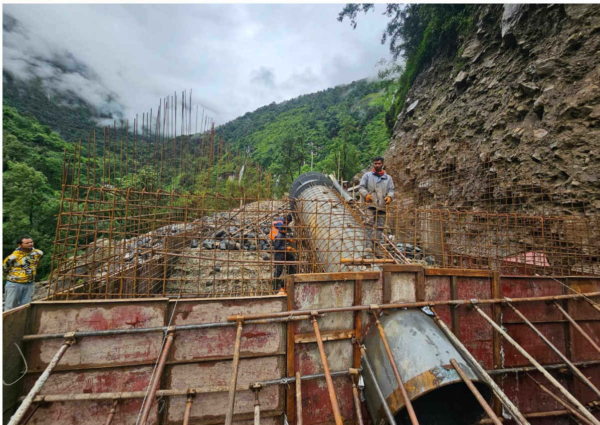
Figure 9: Formwork with support in AB 12
