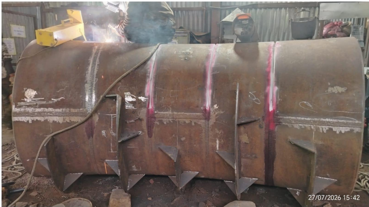
Figure 15: Welding in AB 8 bend in HM workshop
