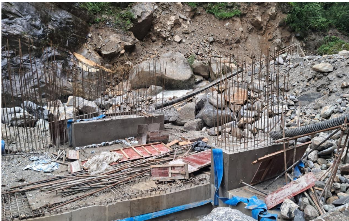
Figure 2: Concreting in wall of Undersluice u/s panel
