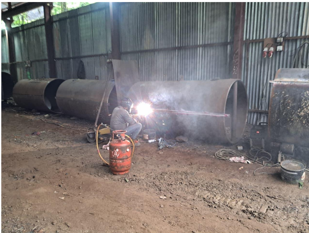
Figure 16: Welding in straight pipe in HM workshop
