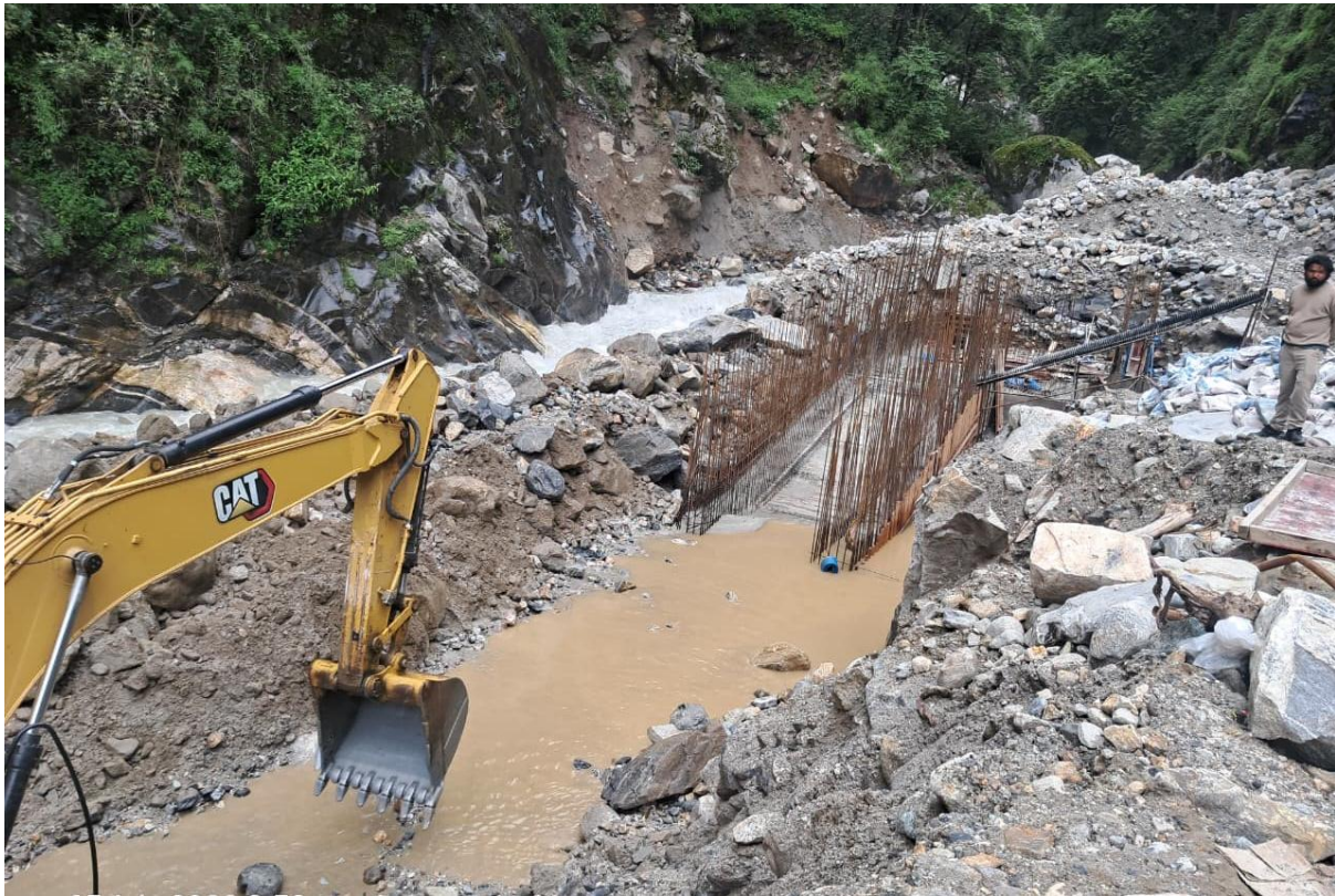
Figure 3: Lowering water level in Undersluice area
