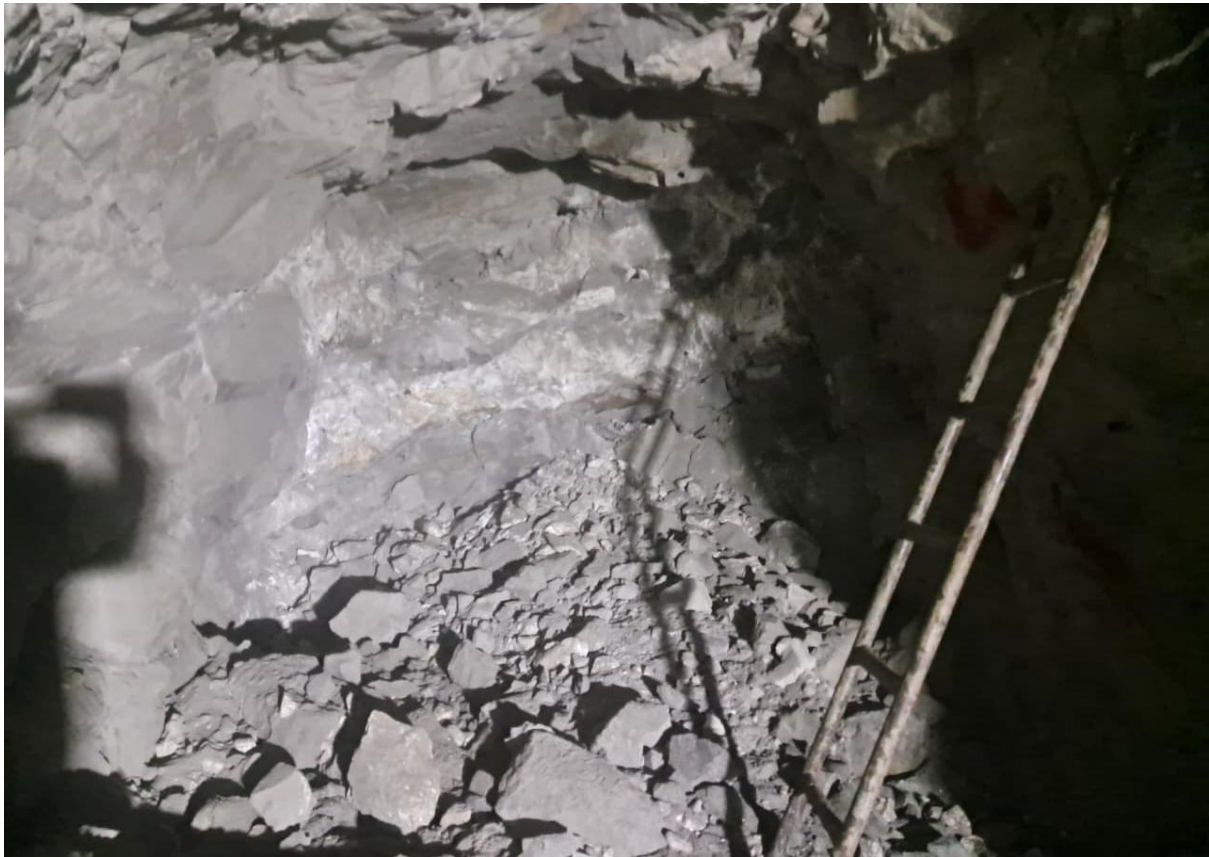
Figure 5: Inlet tunnel face at ch 0+078.10m
